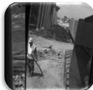
Adjust and clean mirrors; check back-up alarm.
