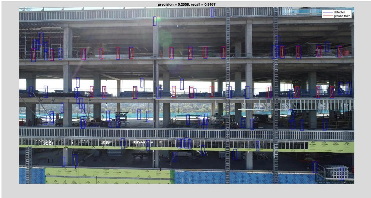
**Figure 12: Visualizations of the guardrail detections using the cascade classifier.**
