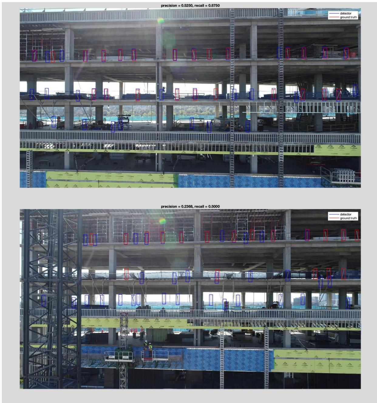
**Figure 14: Final Detection Results on Two Images. The blue bounding boxes are the detected windows and the red ones are the ground truth labels.**
