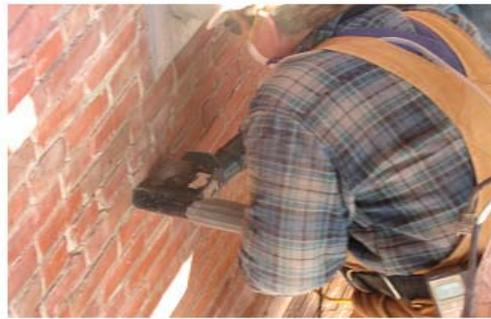
A. Schematic illustration of grinder hood capturing the mortar debris. About 80 cfm of air is exhausted through the grinder. The uncut mortar is intact and directs the mortar debris into the exhaust take-off.
