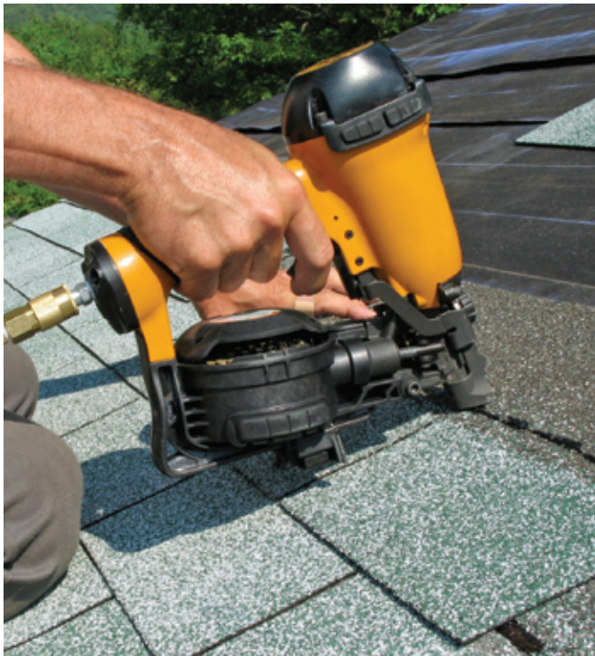
Researchers found nail gun injury rates declined due to increased use of sequential trigger tools and early training of users.
