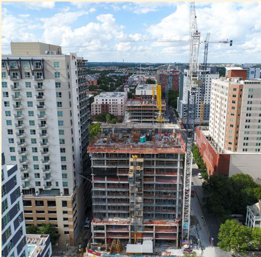
Good safety is critical on tight, complex construction sites.
