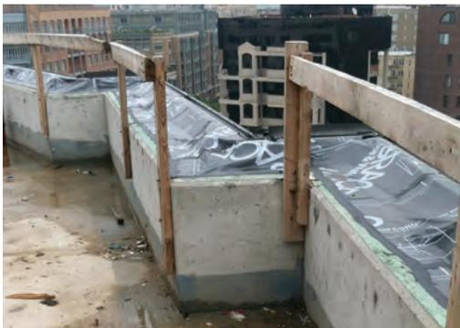
Figure 1: Unprotected roof edge
