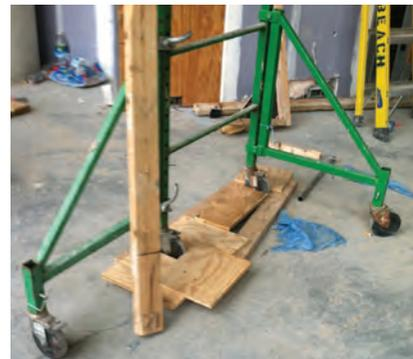
Figure 3: Improperly secured base on mobile scaffolding
