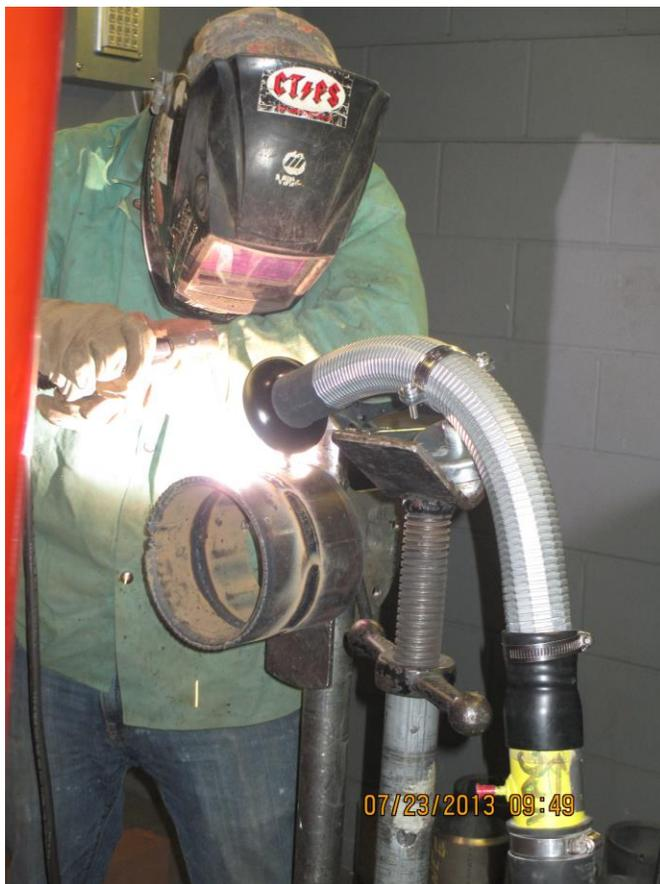
**Figure 3: Welding carbon steel with LEV**
