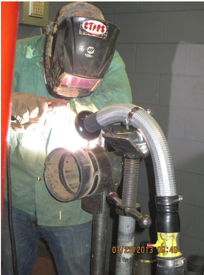
**Figure 3: Welding carbon steel with LEV**
