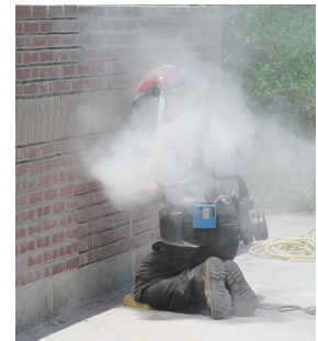
Grinding without LEV
