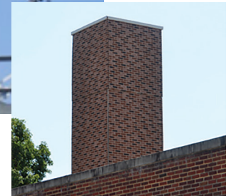
Faux chimney used to conceal 15 panel antennas.
