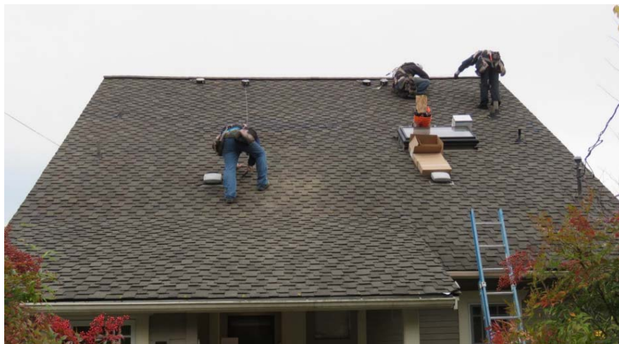
Figure 5. Installing Connections for Mounting System (Picture taken by Chung Ho on 11/17/2016 at Case Study 1)
