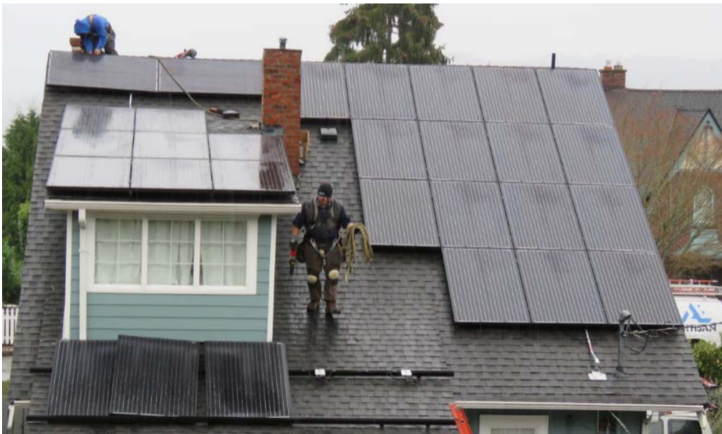
Figure 8. Panel Layout on a Gable Roof with Dormer (Picture taken by Hyun Woo Lee on 11/23/2016 at Case Study 2)
