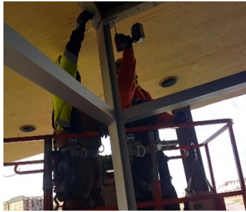
6b- Curtain Wall/Drilling
