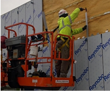
8d- Panel Installation
