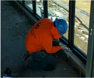
9d- Fill Perimeter with Backer Rod
