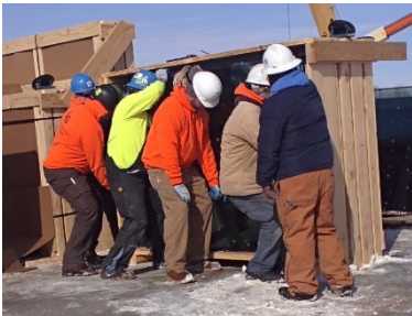
10a- MMH / Lifting
