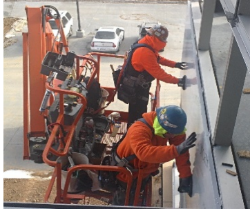
8b - MMH / Placing
