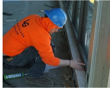
9f- Smooth the Bead with Wet Finger
