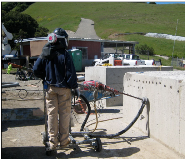
Drill support system with dust-collection.
