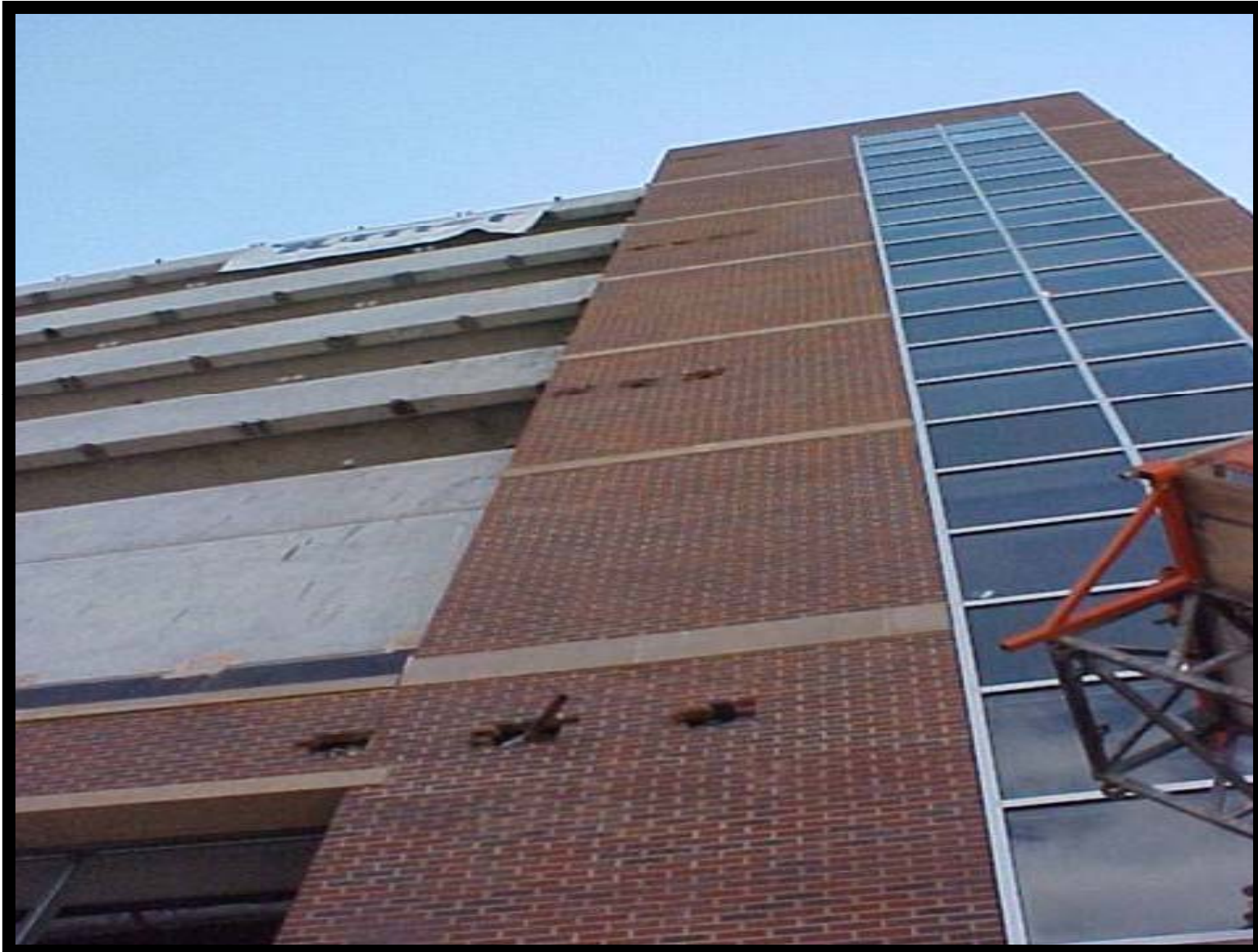
Sections Removed Prior to Accident
