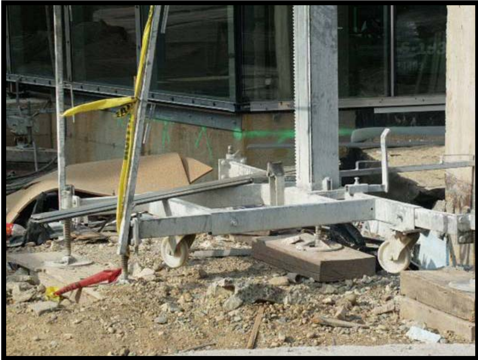
Uneven Surface at Base Support
