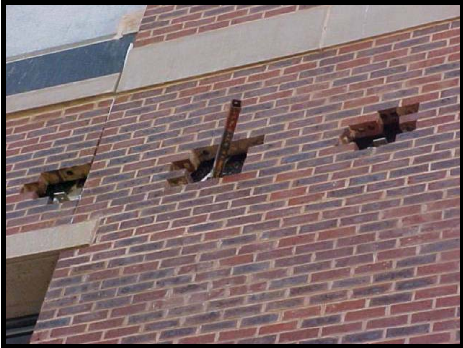
Lower and Last Tie In Removed
