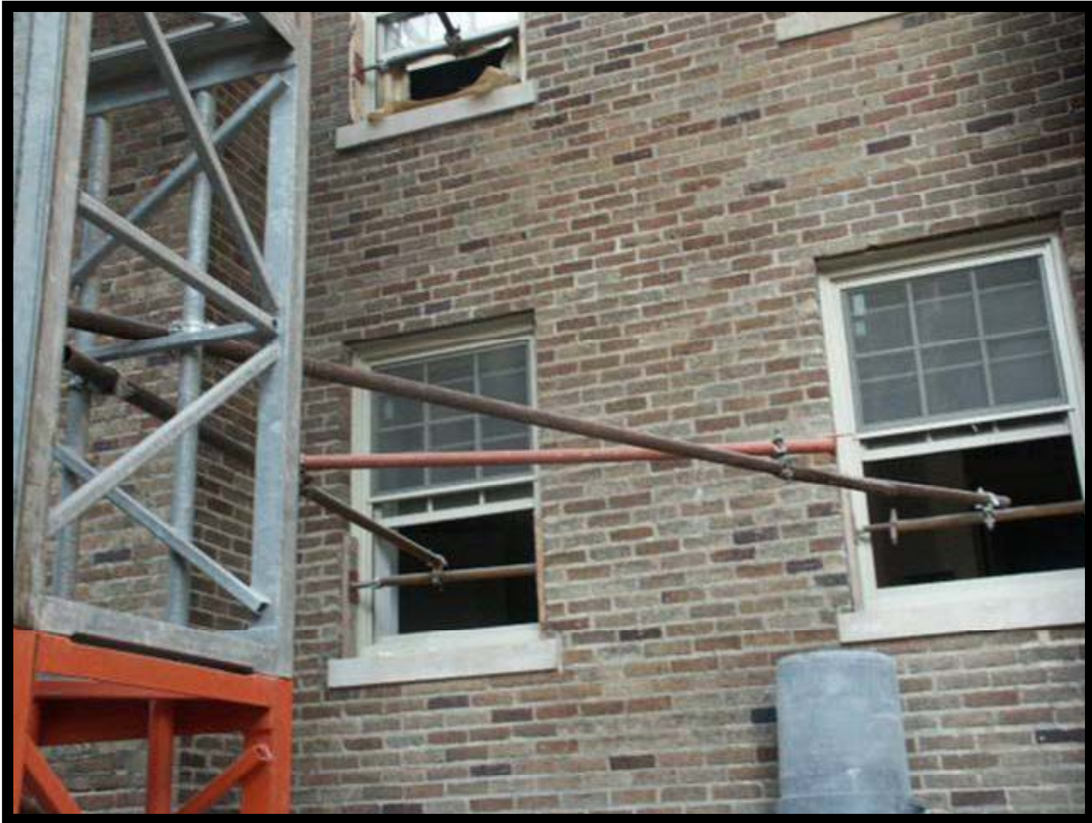
Wedged into Window Openings
