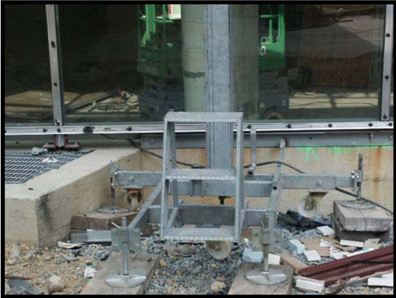
Outriggers and Stabilizers on Sills
