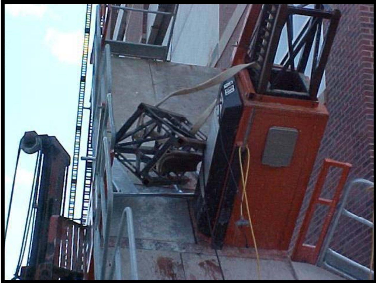
Workers Dismantling Mast Scaffolding
