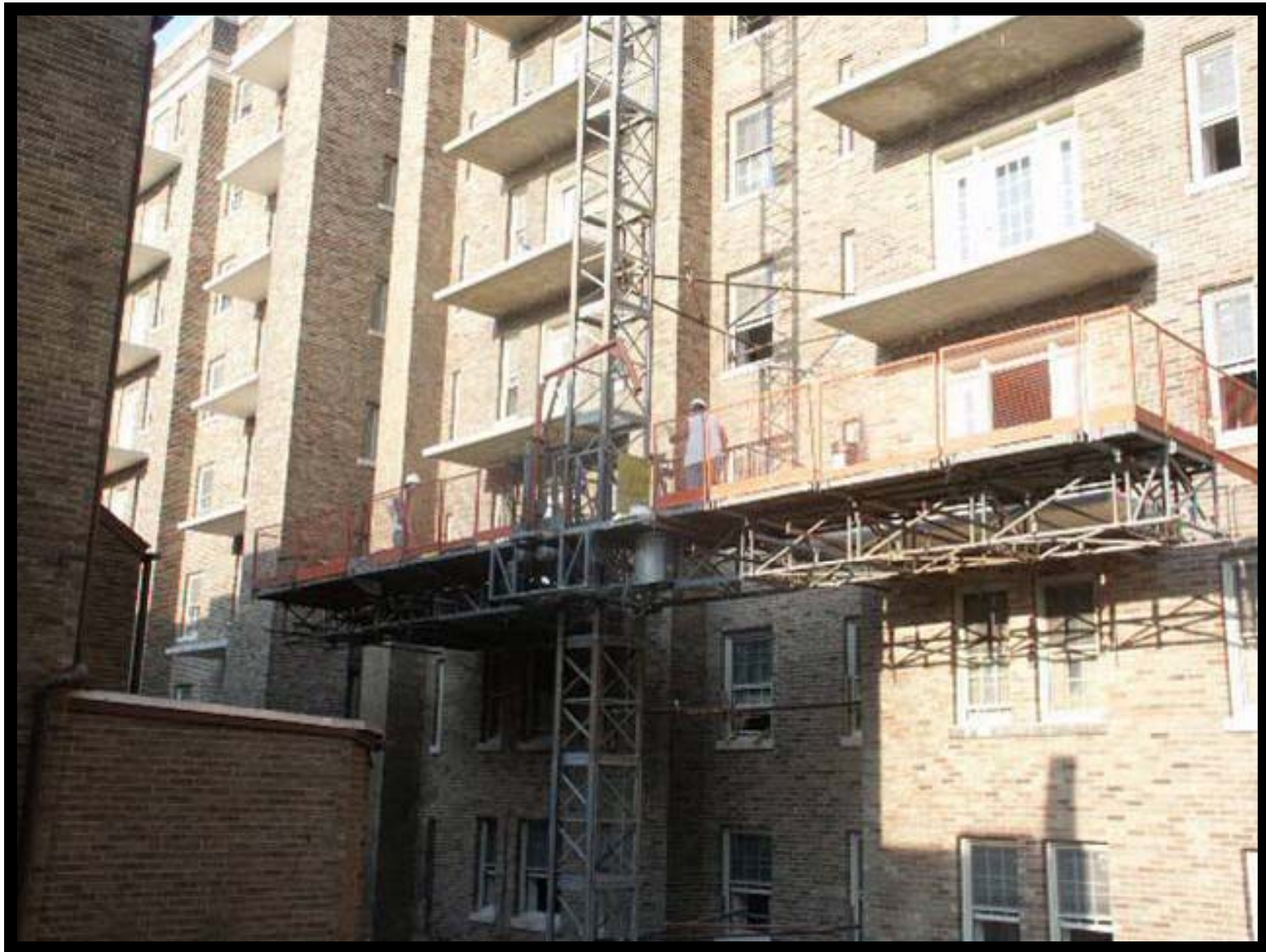
Single Mast with Large Platform
