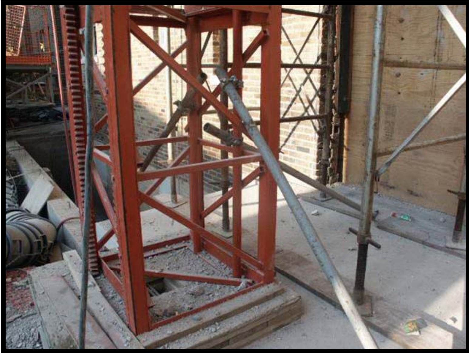
Pole Stabilizers Connected to Mast
