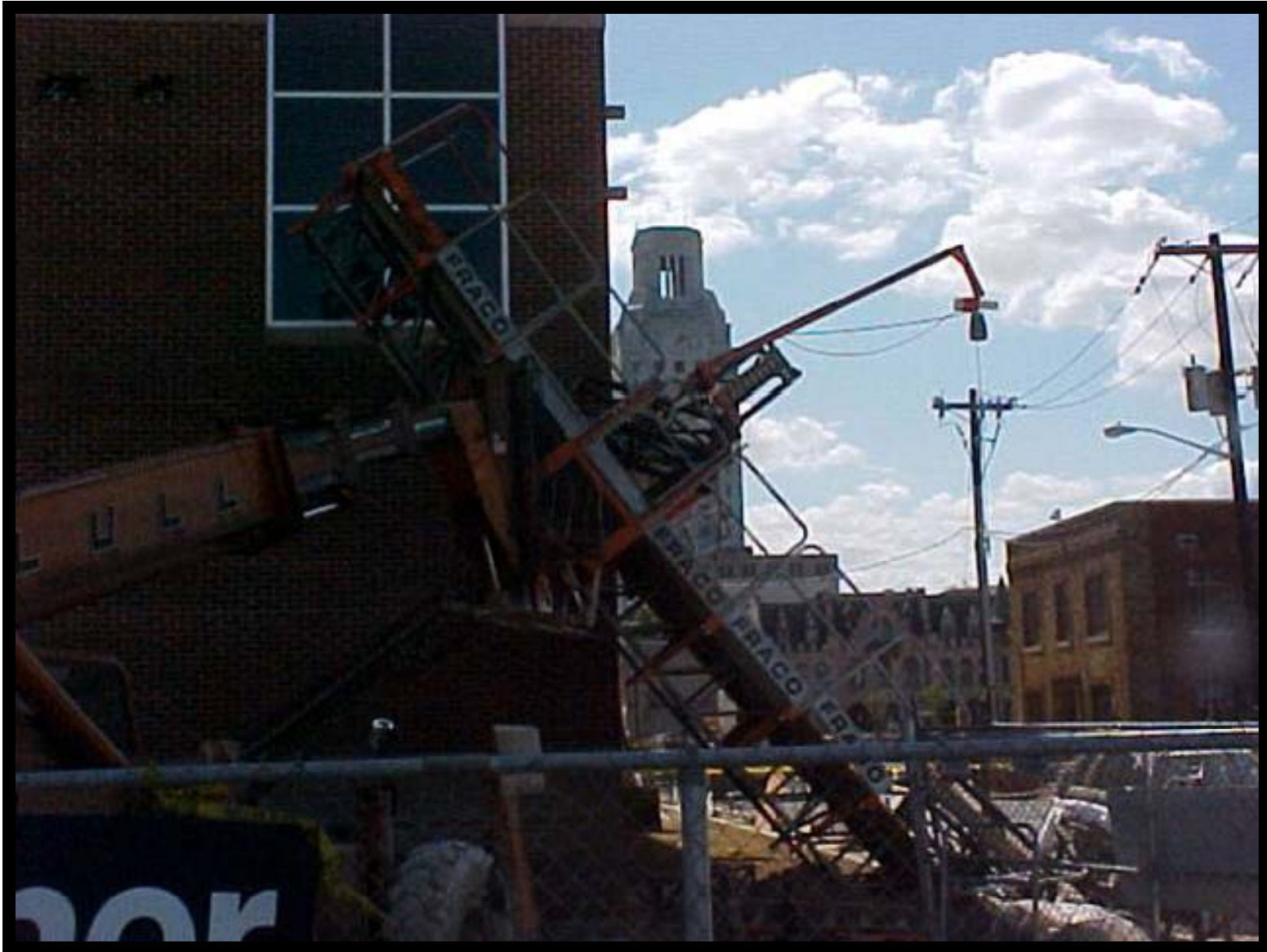
Mast Is Not Bent
