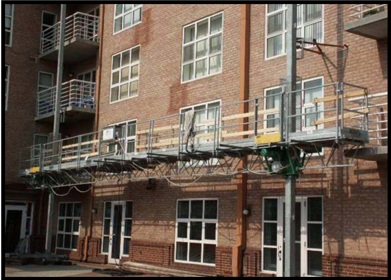
Mast Scaffold Used for Restoration Work
