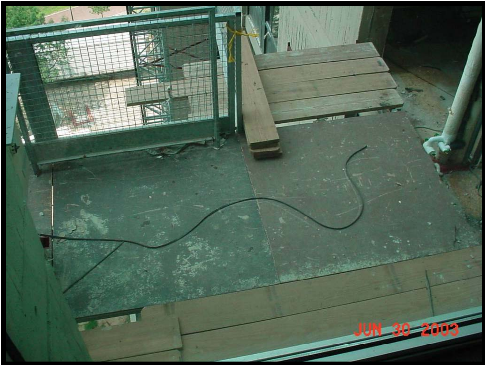
Planking from Which the Worker Fell
