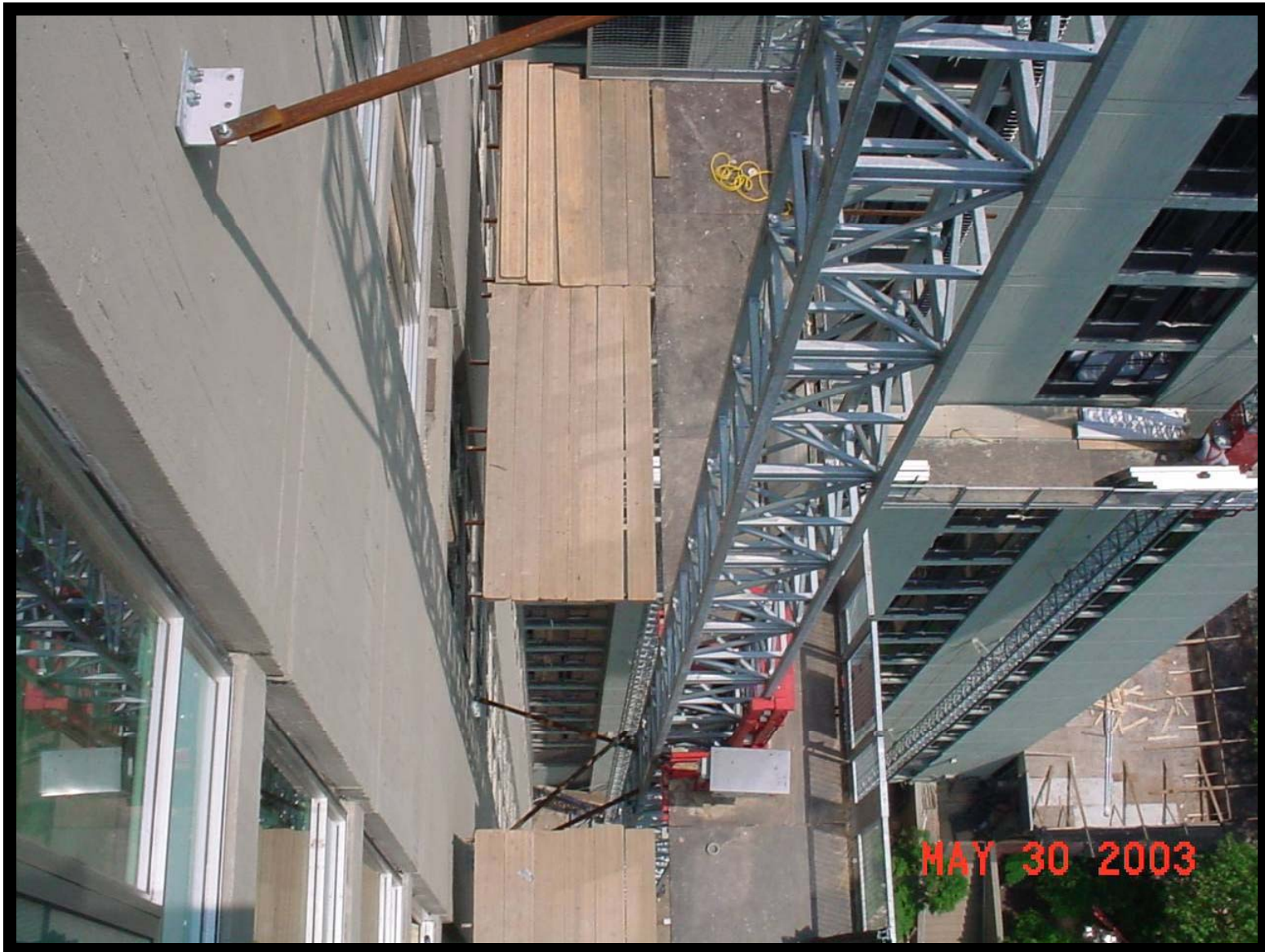
Inadequate Platform Planking
