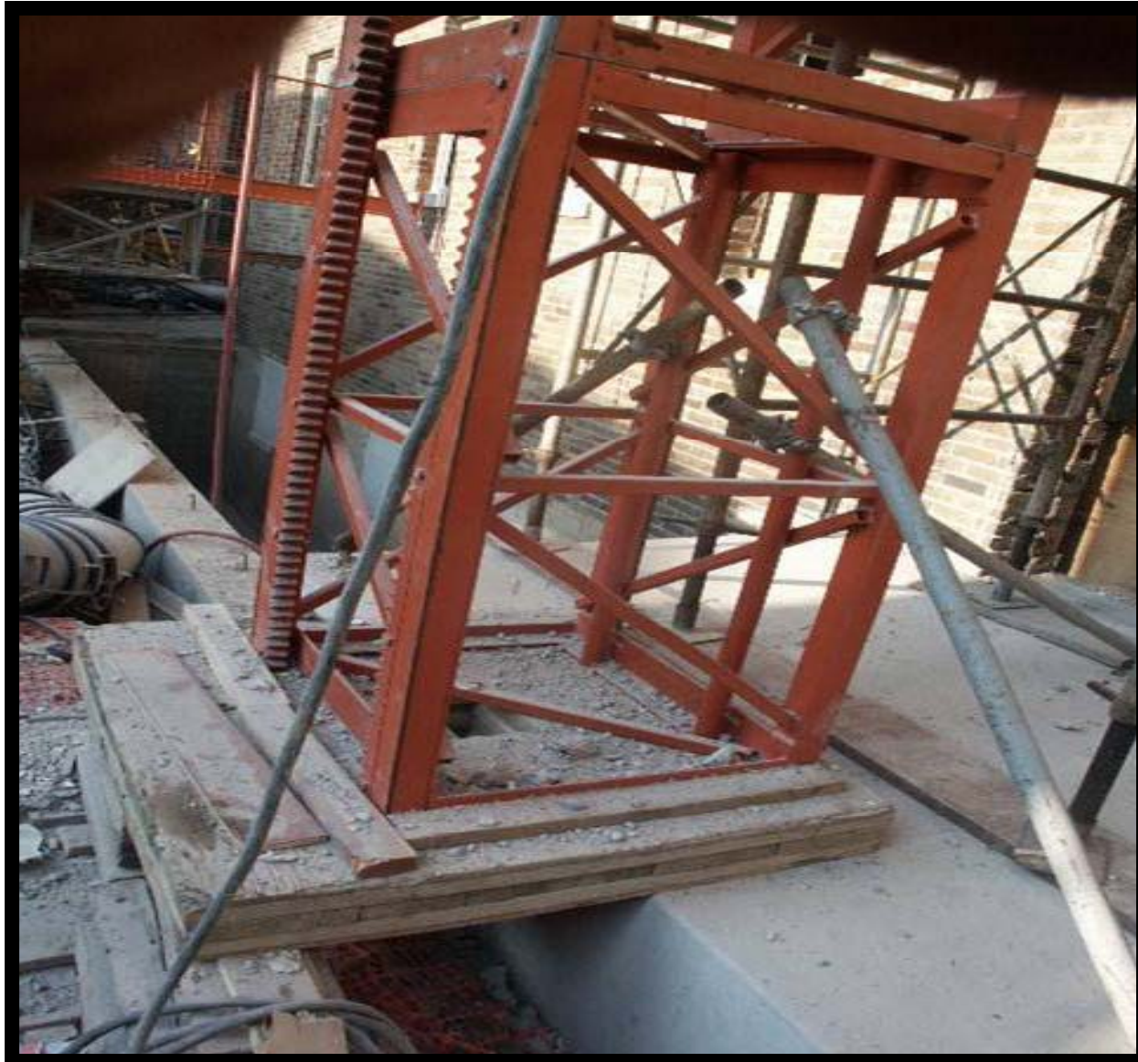
Base Support Bridged over Space
