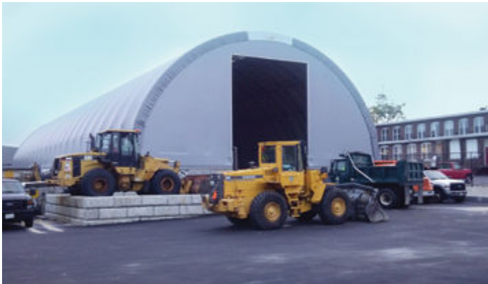
Container foundations are a practical choice for construction sites, because expensive equipment can be locked away safely at the end of the day. (Photo provided by Clearspan Fabric Structures)
